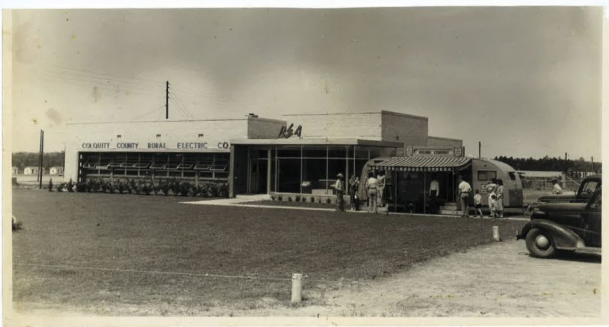
You might recognize this building as Colquitt EMC's old headquarters office (1949 to 2019). Did you know Colquitt EMC used to host the annual meeting on the grounds of the headquarter's office?
